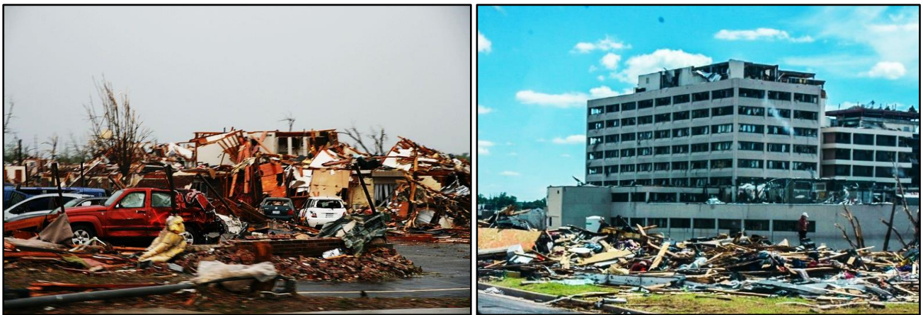
Figure 2. Combined images showing the damage in Joplin following the tornado
